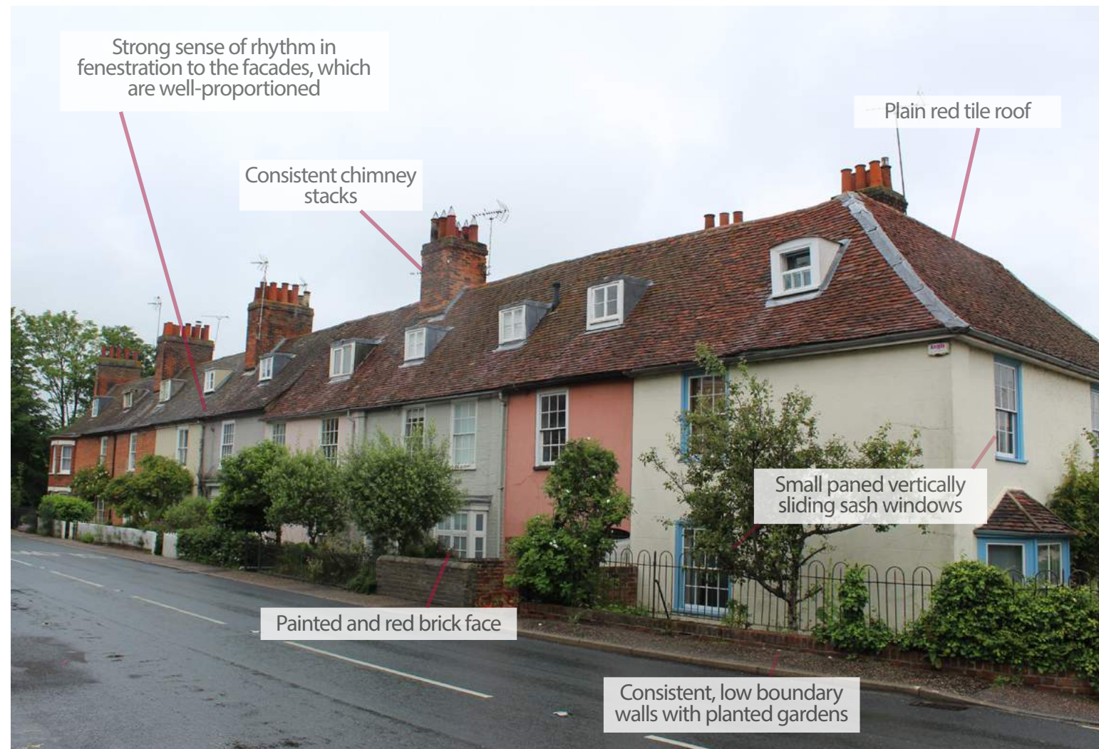
Mistley High Street, Terrace of 8 Cottages (Grade II Listed)
